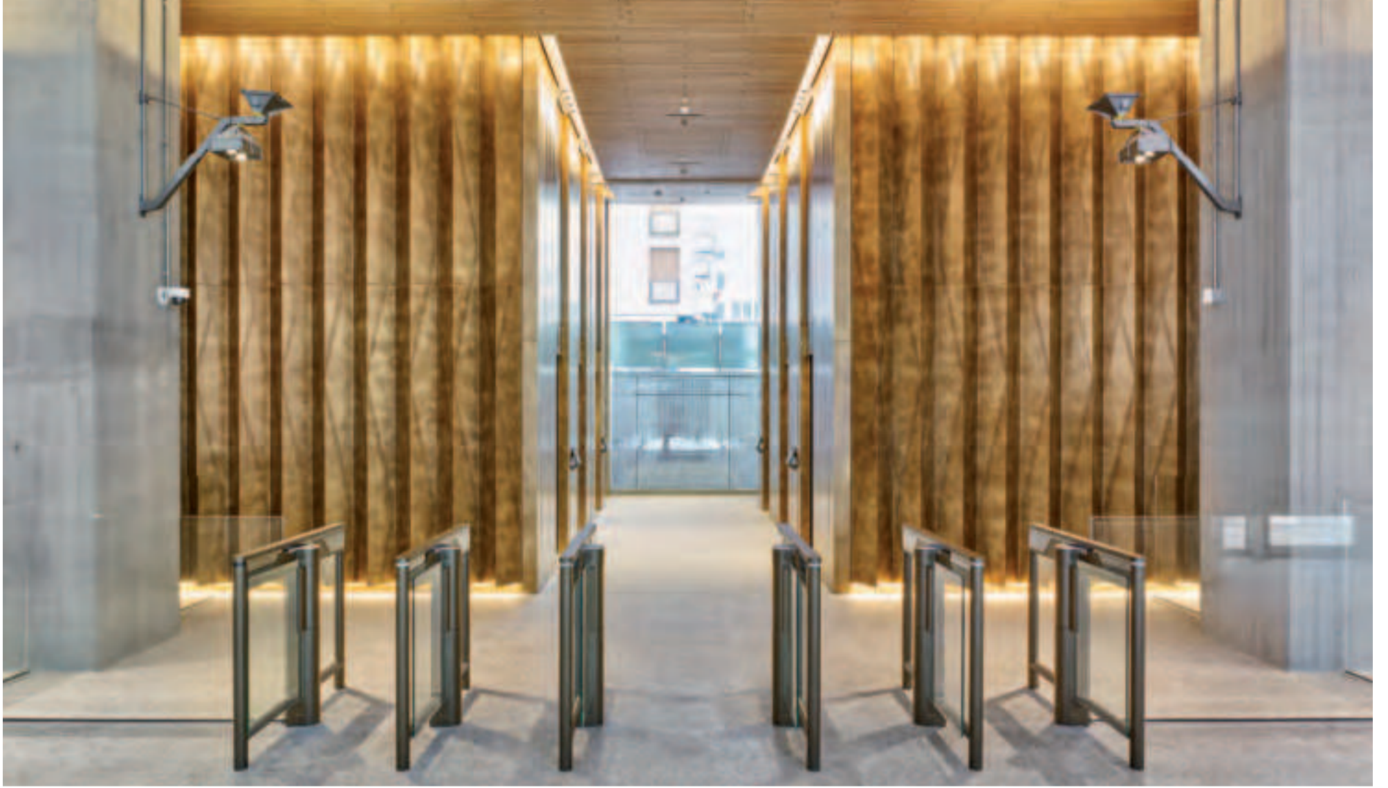
Rivestimento a parete in ottone DeLabré Cladding system in brass DeLabré finishing
